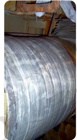
Pipe Wrapping Combinations - Max Temp 170°C / 338°F
