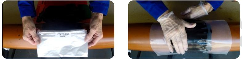
6. Mixing & Application of UPS 19000 RH Standard Resin & Hardener
