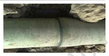
**UPS MiniBlaster** – For the best mechanical surface preparation results, use the UPS MiniBlaster. Ensure all loose material and as much surface contamination is cleaned from the surface. Ensure the surface is wiped with *UPS CLEANER MEK* prior to, and after abrading the surface.
